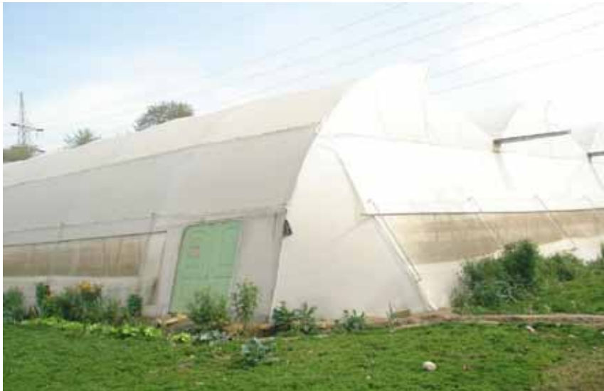
Wrong selection of site
