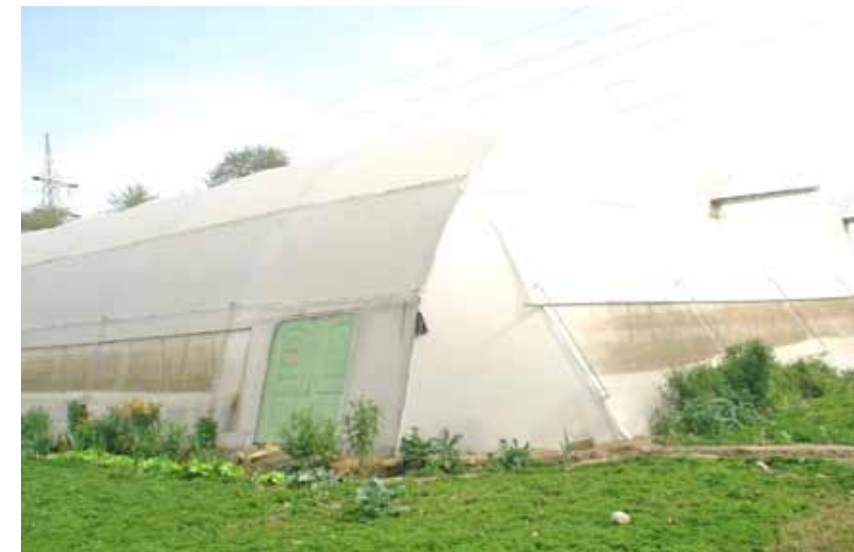
Wrong selection of site
